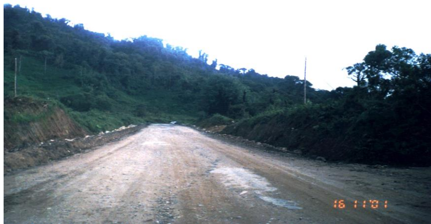
Photograph 7. Road built with material from the natural asphalt mine of the PUNGARAYACU field
