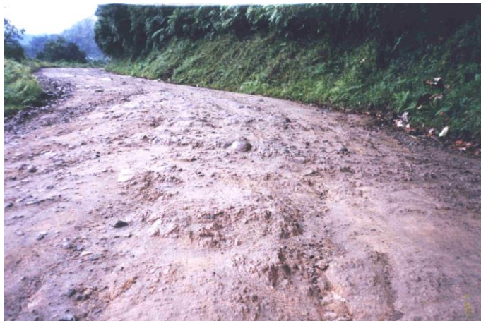
Photograph 2. Swamps in winter on the tracks with a tread layer in asphalt material.
