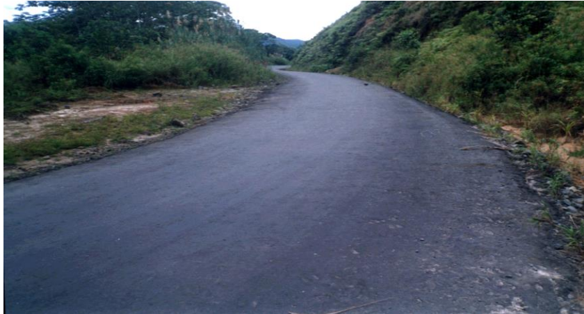
Photograph 6. Road built with material from the PUNGARAYACU field belonging to the Ministry of Public Works (Napo Province - Ecuador)
